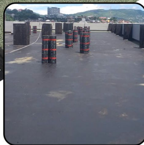
Allow to dry at last 4-6 H
